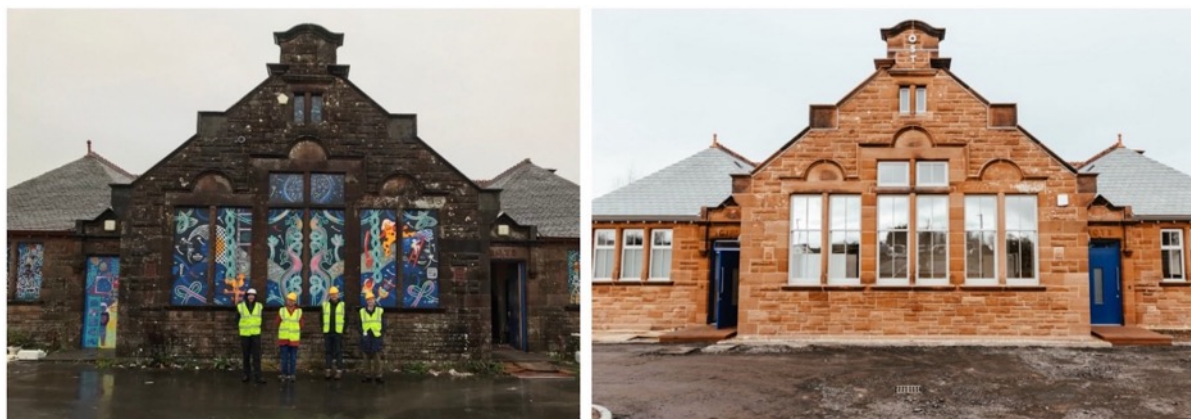
Figure 7 - Thornhill Old School before and after capital works.
