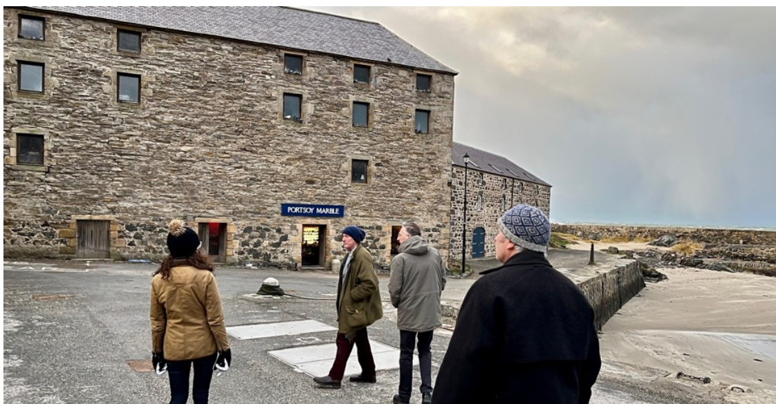
Figure 13 - Cat. A listed Portsoy Harbour Buildings – now owned by NESPT and being supported by AHF grants and the new NLHF funded Heritage Development Trust programme.
